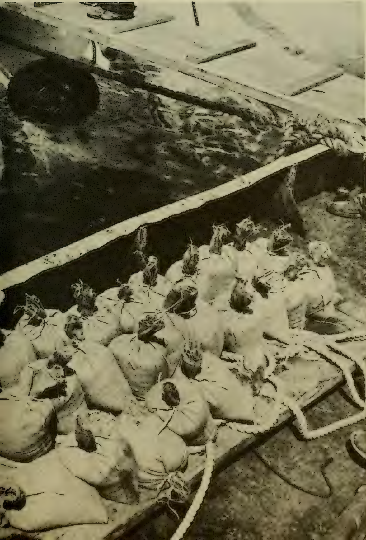
Plate X The iron shot used for ballast
